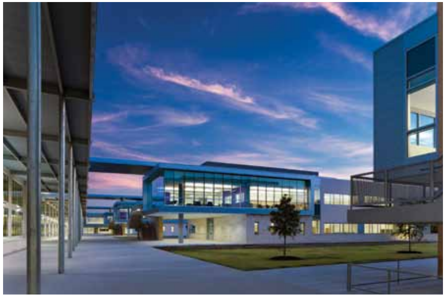
The student courtyard at Cedar Ridge High School in Round Rock, Texas, is flanked by two of the four small learning communities designed for the school, which includes upper-level distributed media center and teacher planning areas. Photo: Charles D Smith Photography
