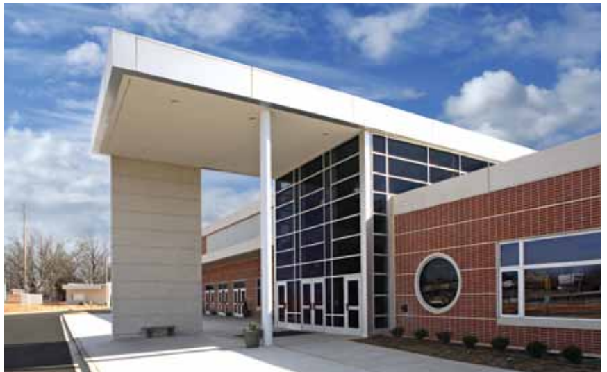
Budget restraints and a search for new delivery methods have brought precast concrete construction to the forefront for many schools. The Carolina High School in Greenville, S.C., was designed by Perkins+Will with a total precast concrete system of load-bearing wall panels and double tees. The project won the award as Best School Design in the 2007 PCI Design Awards competition. Design Architect: Perkins+Will. Local Architect of Record: Craig Gauden Davis. Photo: Michelle Gunning
