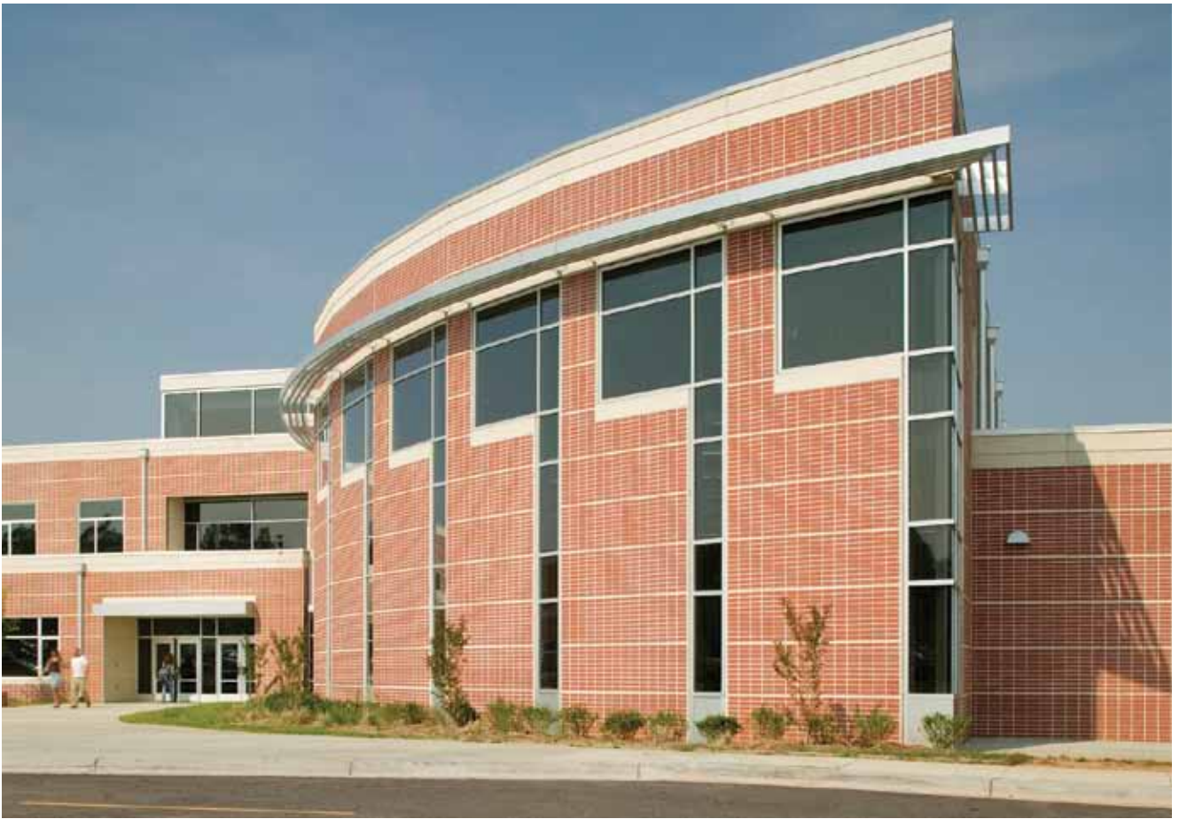
Travelers Rest High School in Travelers Rest, South Carolina, welcomes students with an exterior featuring precast concrete exterior wall panels accented with thin brick. Design Architect: Perkins+Will. Local Architect of Record: Craig Gaulden Davis. Photo: Creative Sources Photography
