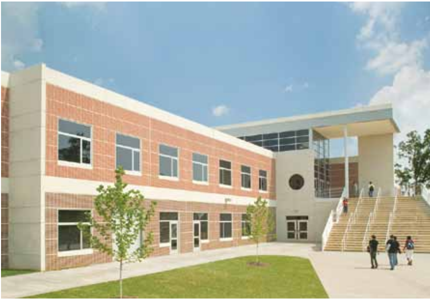
The Carolina High School in Greenville, South Carolina, shows that precast concrete can simulate the traditional look of brick that administrators want to retain while providing more contemporary benefits of an engineered material. Design Architect: Perkins+Will. Local Architect of Record: Craig Gaulden Davis. Photo: Creative Sources Photography
